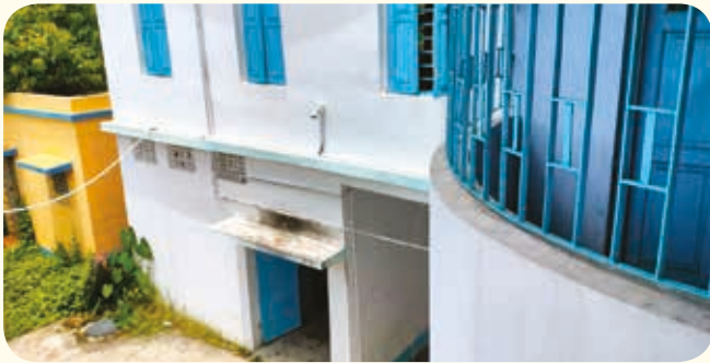
Restoration of school building and facilities at Sarengabad High School (H.S.).
